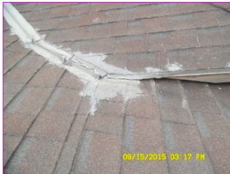
ASPHALT SHINGLES General Condition
