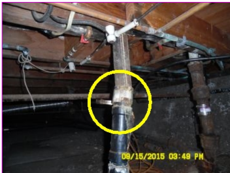
connector clamp broken
