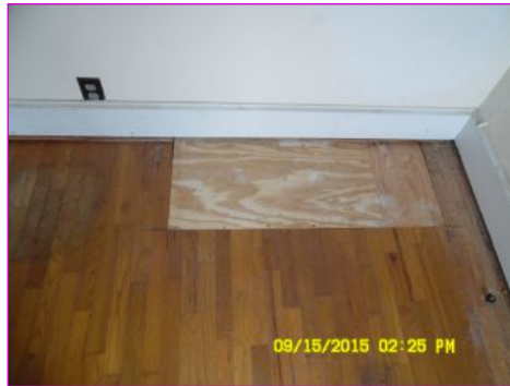
Temporary floor repair
