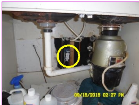
Outlet not secure, no plate.
