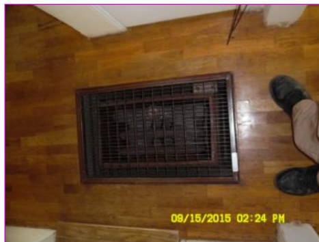
Original floor furnace
